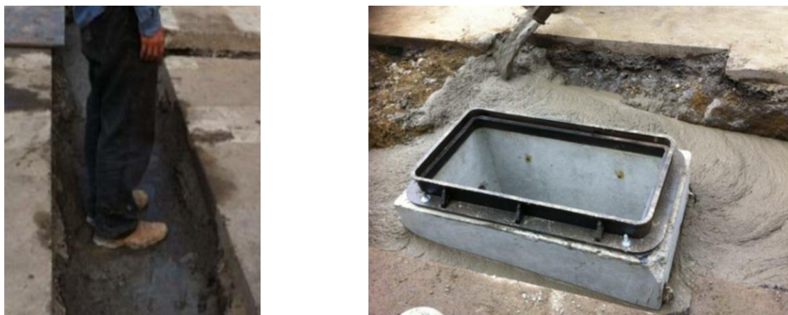
Figure 4.6.2.5-4 (left) After CLSM backfilling, ask 60kg staff to stand on it for 5 minutes to test, (right) Diagram of Backfilling CLSM to Pipe Trench (for reference only)
