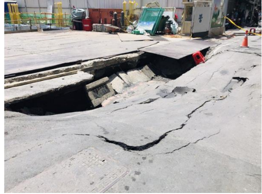
Figure 4.6.2.5-2 (left) Ground Cracking (right) Backfill Material Structural Damage (for reference only)
