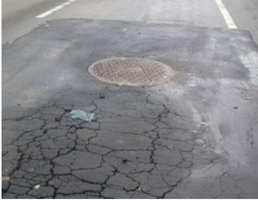
Figure 4.6.2.5-2 (left) Ground Cracking (right) Backfill Material Structural Damage (for reference only)
